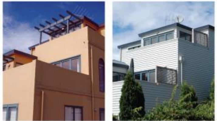
Before & After Cladding
