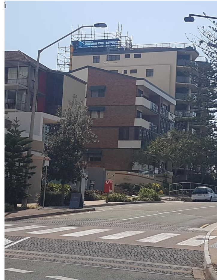
Works as at Thursday 15 th February 2018
