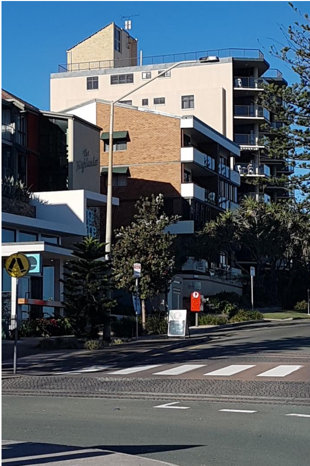
Before works commenced
