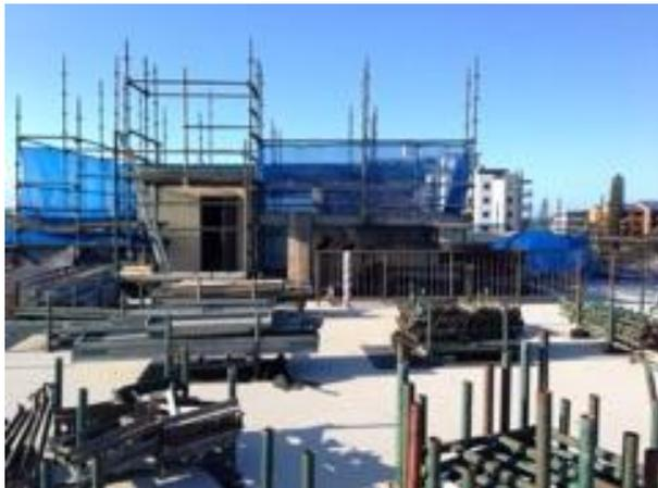
General view on rooftop, looking North towards new work, some scaffolding partially dismantled and palletted, ready for removal by crane.
